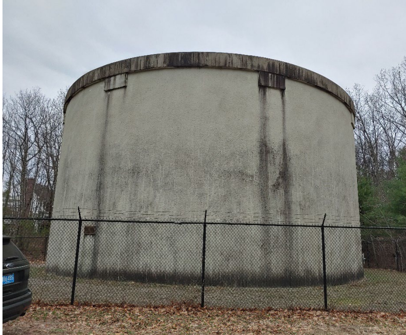
Picture 1-6 Bucks Hill Storage Tank
