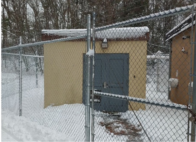
Picture 1-3 Well 3 Building Exterior
