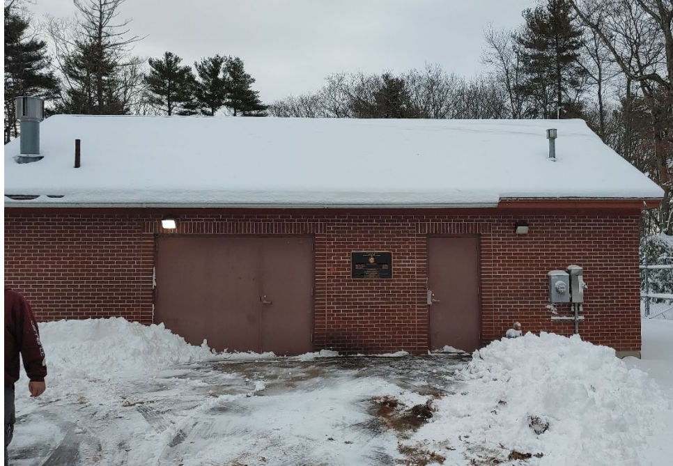
Picture 1-4 Treatment Facility #5 Building Exterior
