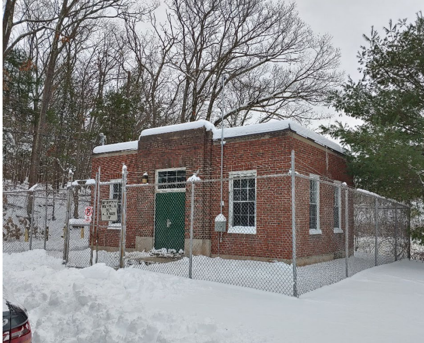
Picture 1-2 Well 2 Building Exterior
