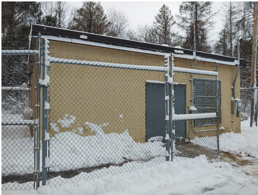
Picture 1-1 Treatment Facility #3 Building Exterior
