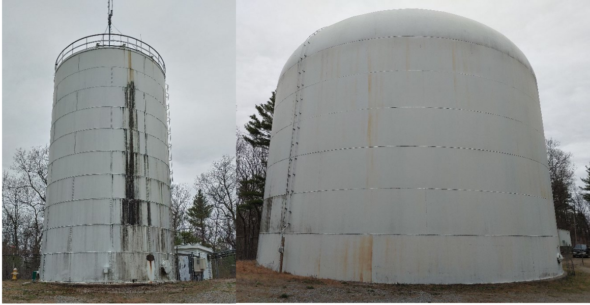
Picture 1-7 Knuckup Hill Storage Tanks (250,000 gallon left, 1,500,000 gallon right)
