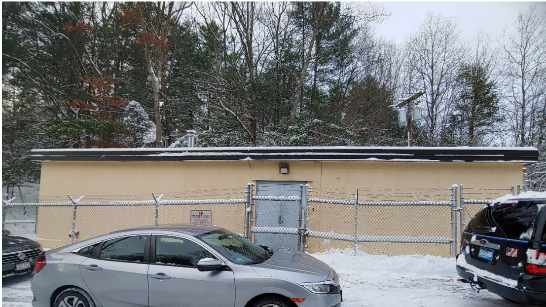
Picture 1-5 Treatment Facility #4 Building Exterior
